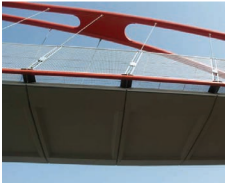
Figure 18: Suspension of the deck on the arches
