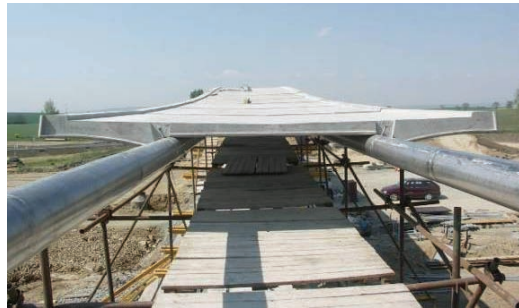
Figure 9: Precast segments on external cables
