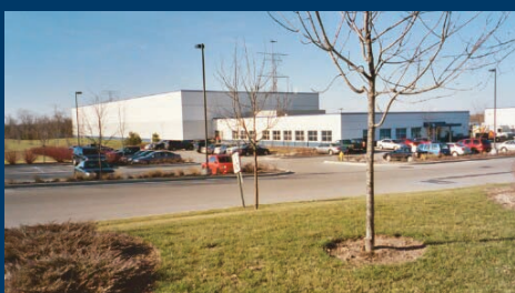
Figure 1 – a typical regional shipping and receiving warehouse in northern USA
