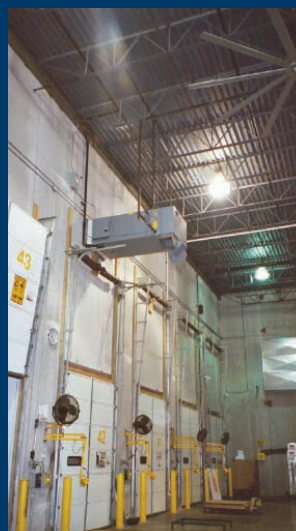
Figure 2 – wall-mounted furnace and large ceiling fan (top right) inside warehouse
