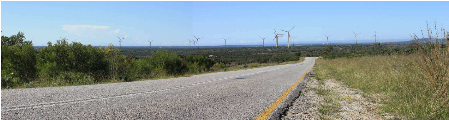
Project as seen from the south of the N2 inside the Coega IDZ
