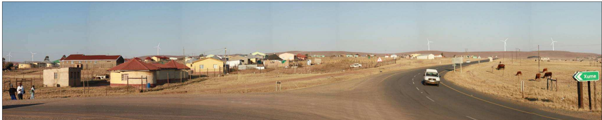
Project as seen from the R409 between Tsomo and Nqamakwe
