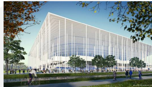
New Bordeaux Stadium (with Vinci)
