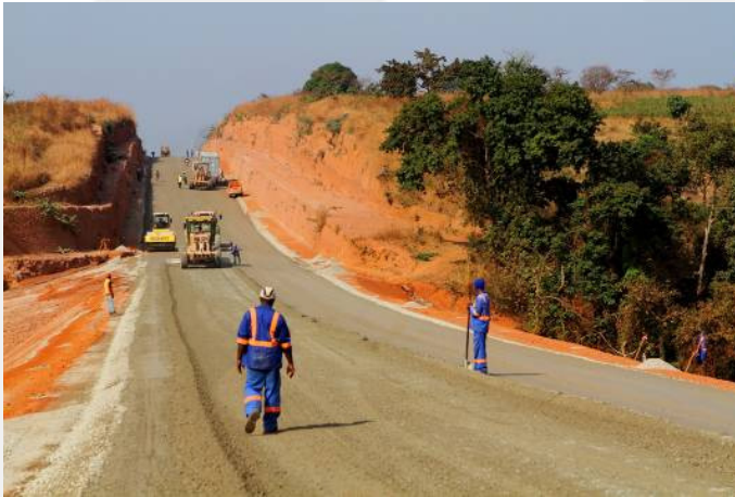
Road in Cameroun – Razel-Bec
