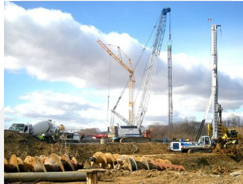
Foundations – Franki Sud
