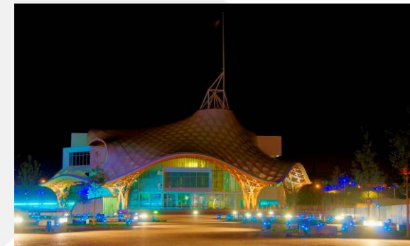
Centre Pompidou Metz
