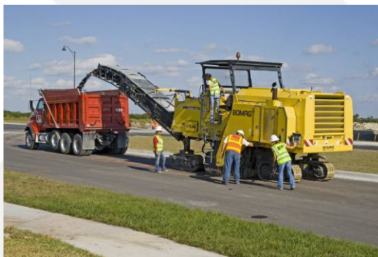
Cold milling machine - Bomag
