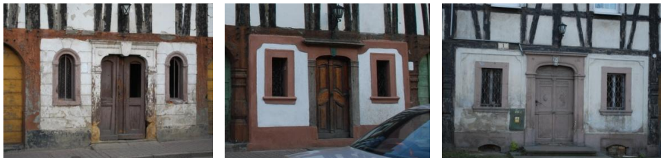
Fig.43. Examples of entrances to typical umgebinde houses [Autho's photographs]
