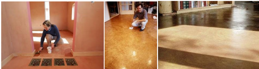
Fig.73. Examples of contemporary clay floors impregnated with natural waxes and linseed oil.
