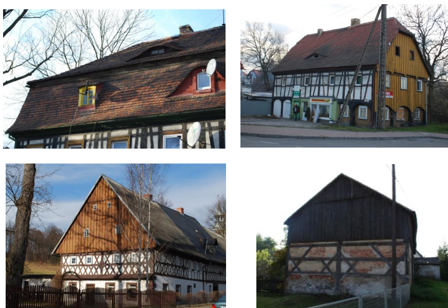
Fig. 39. Photographs illustrating the variety of roof forms in Upper Lusatia [ Author's photographs]
