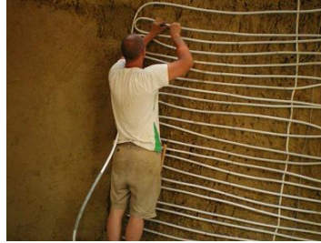
Fig. 84. A photography illustrating the process of heating pipes installation (N).
