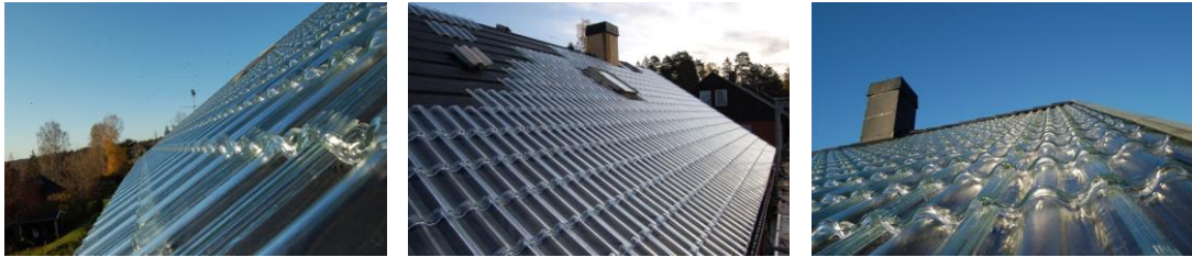
Fig.81. Examples of solar tiles that may be used as photovoltaic panels in the designed house (R)
