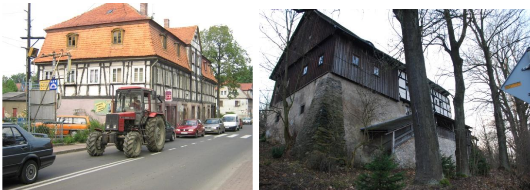
Fig. 31. Photographs of bigger umgebinde houses in Bogatynia and Miskowice [Author's photos]
