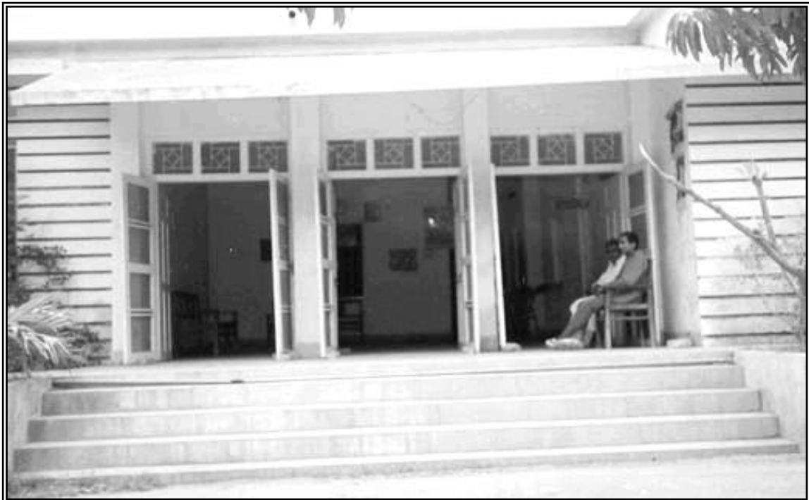
Plate 3.4: View of village hospital
