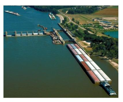
The maximum lift is 10.5 feet with an average lift of 6.55 feet. It takes approximately seven minutes to fill or empty the lock chamber.
