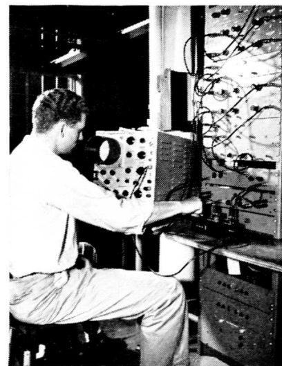
Electrical performance test of Switching Transformer, Union Street Plant, North Adams, Mass.
