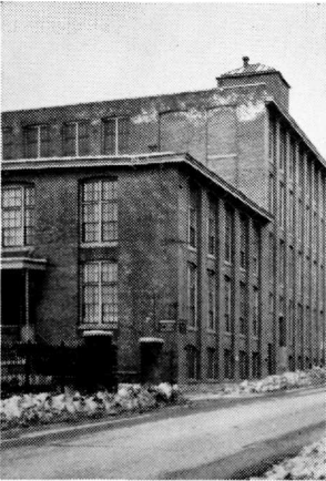
UNION STREET PLANT North Adams, Massachusetts
