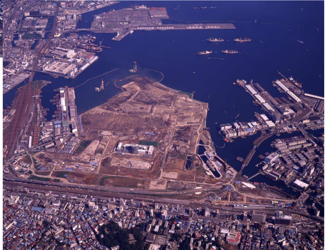
Reclamation Works almost Completed October, 1987
