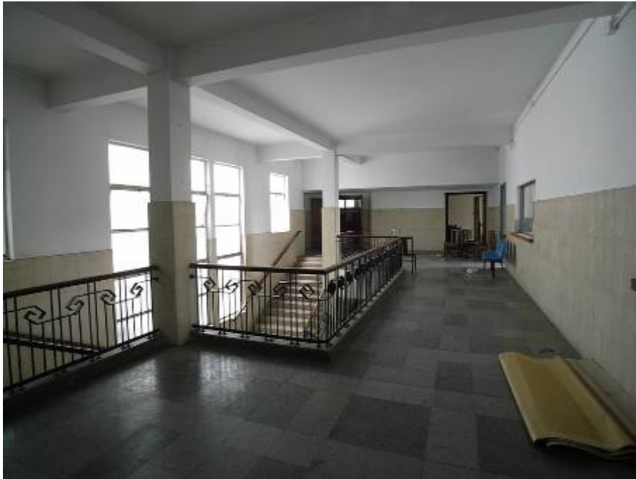
View of public lobby at upper floor of Former Fanling Magistracy
