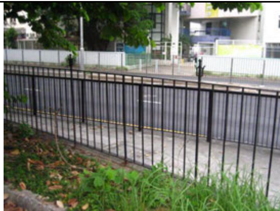
2.1) Simple ornamented iron fencing at the boundary facing Jockey Club Road
