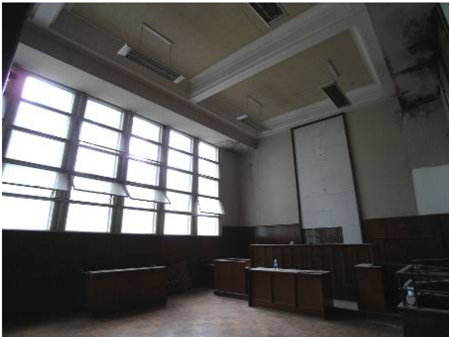
View of Courtroom No.1 of Former Fanling Magistracy
