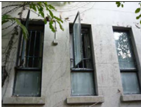
1.14) Regularly spaced window openings with metal window frame, protruding window sills and metal bar/ mesh behind
