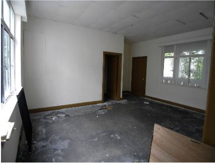
View of Magistrates' chamber at upper floor of Former Fanling Magistracy
