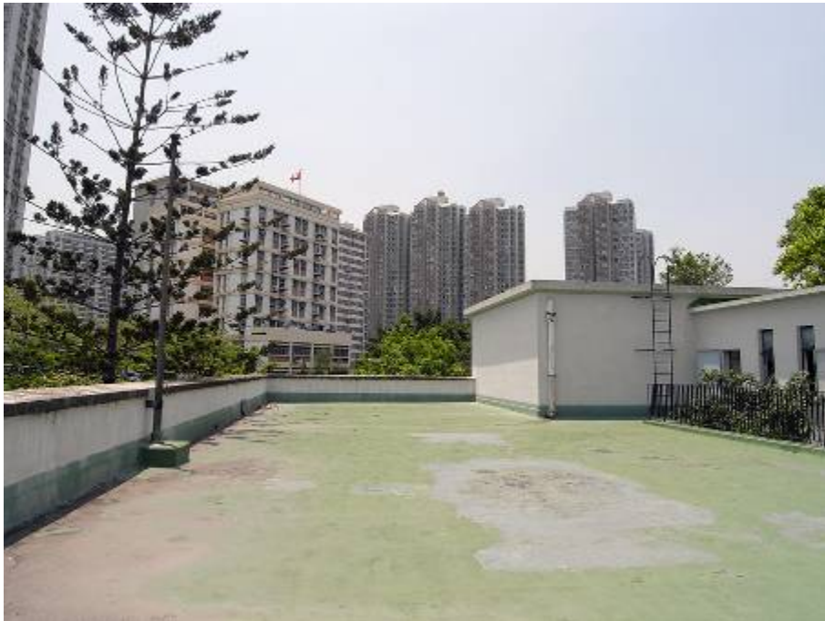
View of flat roof of Former Fanling Magistracy
