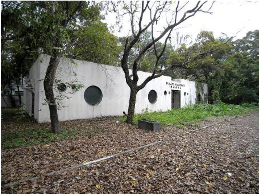
View of main façade of Annex Court Building
