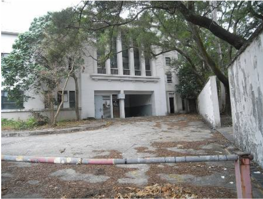
View of north façade of Former Fanling Magistracy
