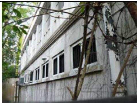
1.14) Regularly spaced window openings with metal window frame, protruding window sills and metal bar/ mesh behind
