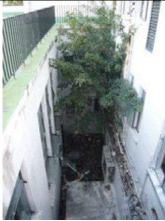
1.21) Light well with narrow windows to atrium
