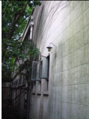
1.14) Regularly spaced window openings with metal window frame, protruding window sills and metal bar/ mesh behind
