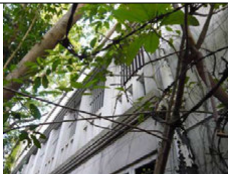
1.15) Featured parapet of 1/F semi-outdoor corridor
