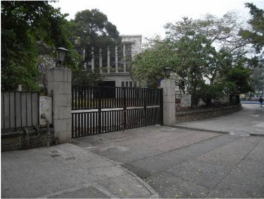
View of vehicular entrance gate at Sha Tau Kok Road – Lung Yeuk Tau
