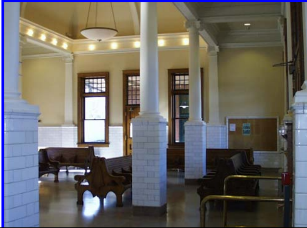
AFTER: New terrazzo, refinished benches and cleaned tile work now reflect light into the rotunda dome.
