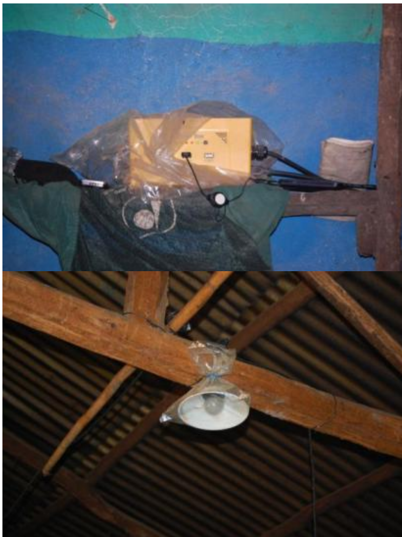
Picture 22: The Power box and lamp of the SHS. The family keeps it in a plastic bag to protect it from smoke and dust.
