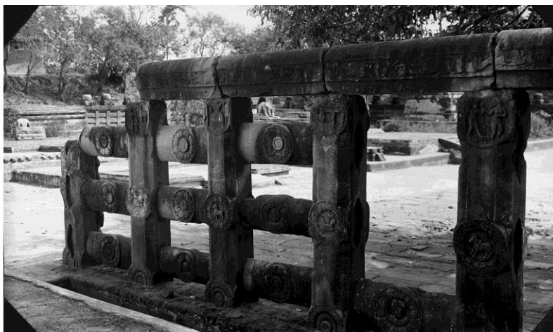
Figure 10. Stone railing at Bodh Gaya, Bihar, India, constructed in a manner similar to wooden railings. From the Marshall photograph collection, held at the Oriental Museum, Durham University (Volume 41, #3234).
