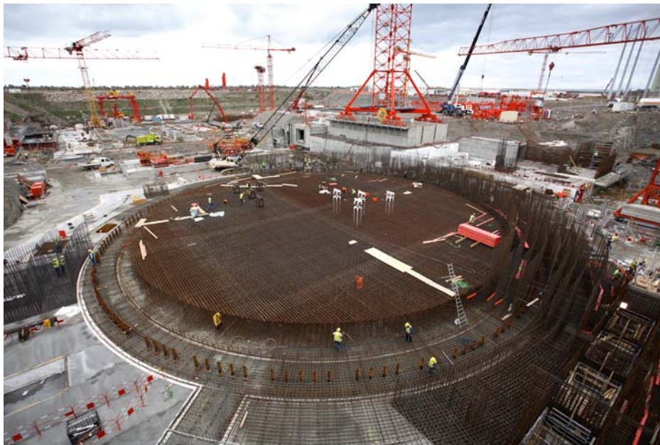
The EPR site in Flamanville in December 2008 (EDF Médiathèque – Alexis MORIN)
