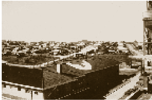
Nurses quarters viewed from the Administration Building construction, 1944. 29
