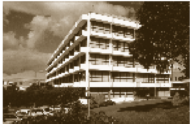
The new Multistorey Wing. 53
