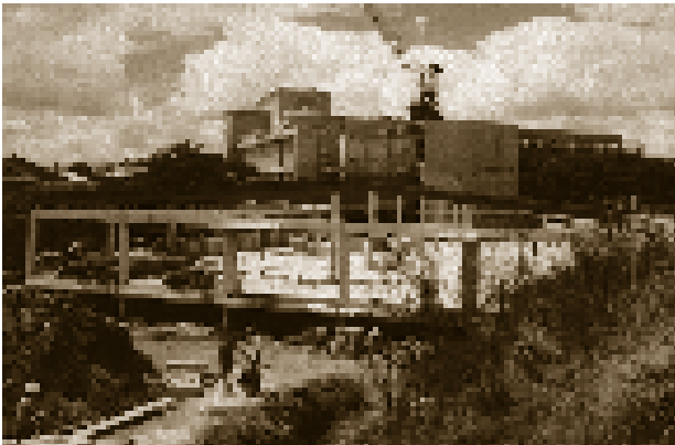
Outpatients Clinic construction, 1974. 49
