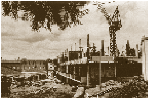
Multistorey Wing construction, 1980. 52
