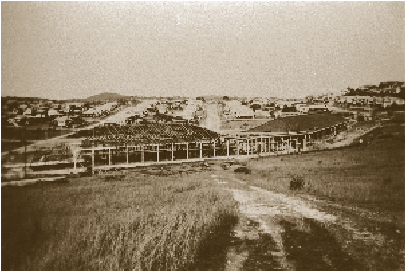
Construction of the wards on three terraces. 9
