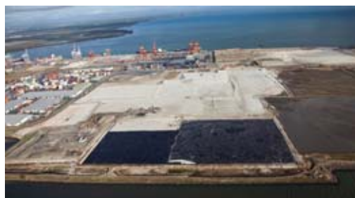
The Future Port Expansion area, where the award winning ground improvement trials were undertaken.
