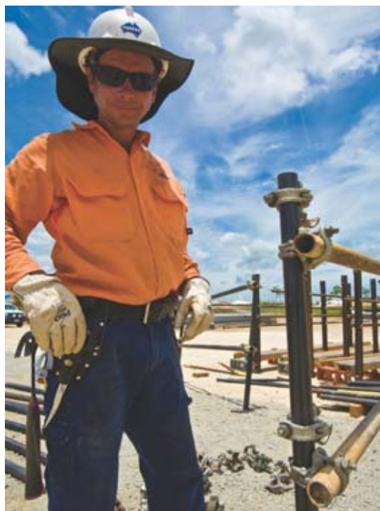
The Thiess team has helped reduce congestion on Townsville’s busy streets through the Townsville Ring Road Project.
