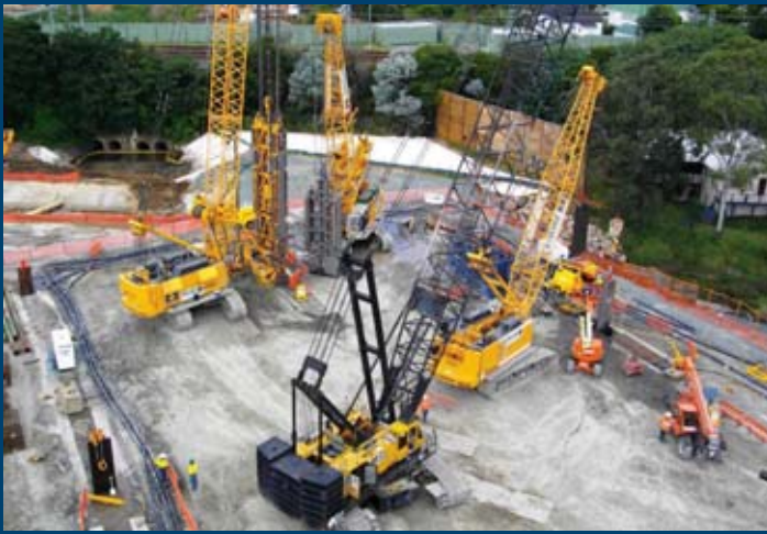
Airport Link Tunnel – Brisbane Diaphragm Walls and Barrettes
