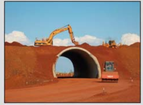
Bridge-Plate arch, Yandi, WA
