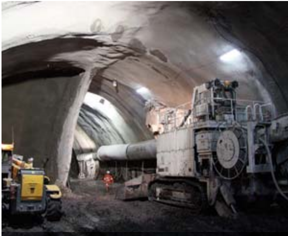
Brisbane Airport Link, Northern Busways and Airport Roundabout Upgrade
