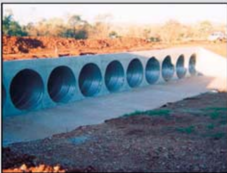
STILCOR 2.4m dia. CMP culverts, WA
