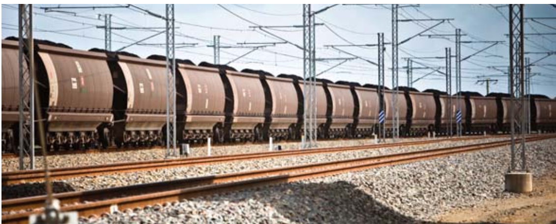
QR Network's COALRail Infrastructure Program is supporting the expansion of the Central Queensland export coal industry.
