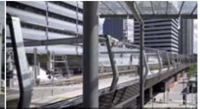
Chatswood Transport Interchange, NSW
