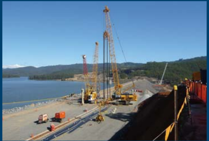
Hinze Dam – Queensland Cut-Off Wall up to 50 metre depth
