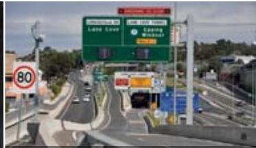
Lane Cove Tunnel, NSW
