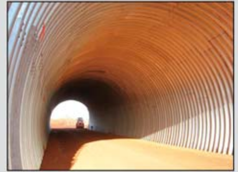
Bridge-Plate arch, Yandi, WA
