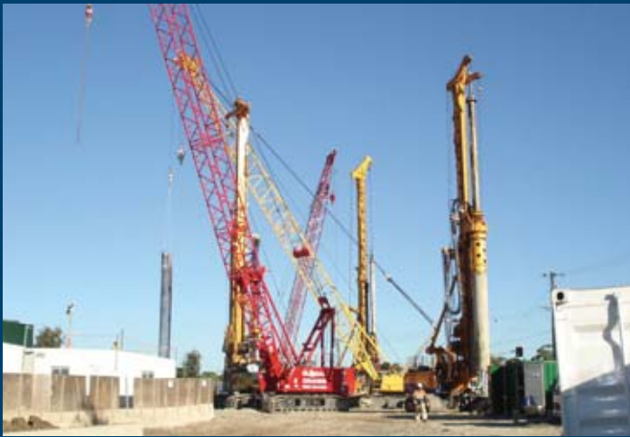
Airport Link Tunnel – Brisbane Secant and Bored Piles
