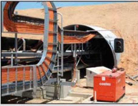
Conveyor tunnel, Wilpinjong, NSW
