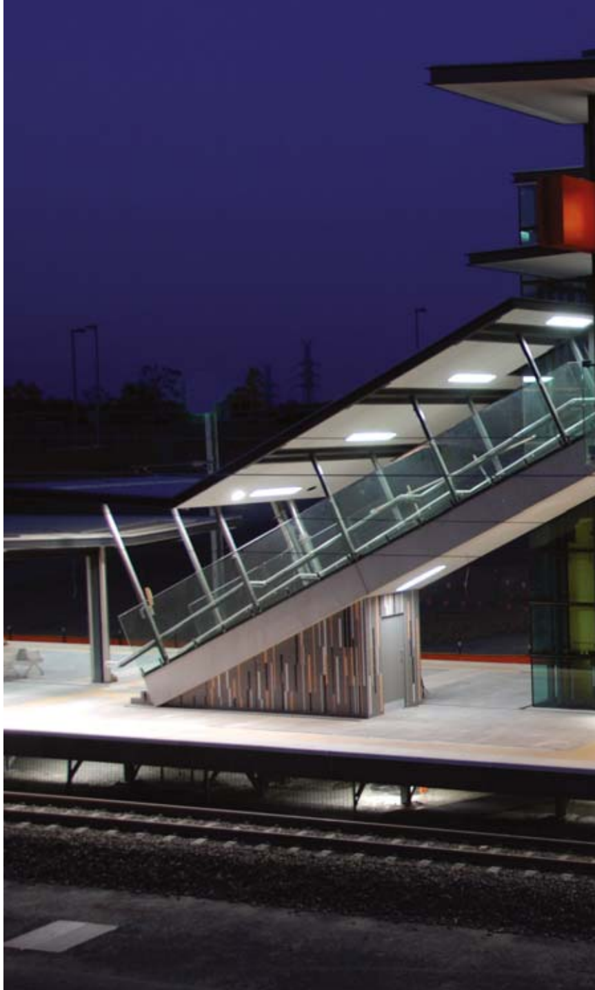
The completed Varsity Lakes station which opened in December 2009
