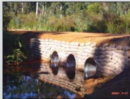
ALUCOR 1.2m dia. CMP culverts, WA
