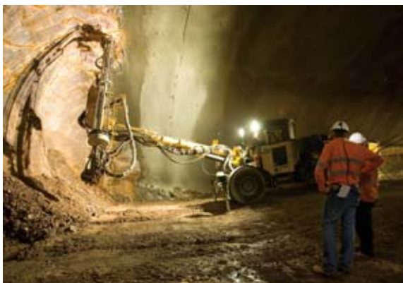
Tunnelling on the Airport Link Project.
