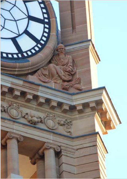
Completed works to the Clock Tower at Central Station.
