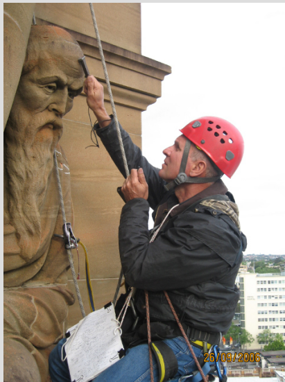
Stone-by-stone analysis during abseiling of Clock Tower (2006)
