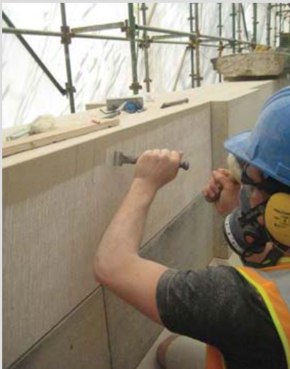
Stonework retooled after indenting.
