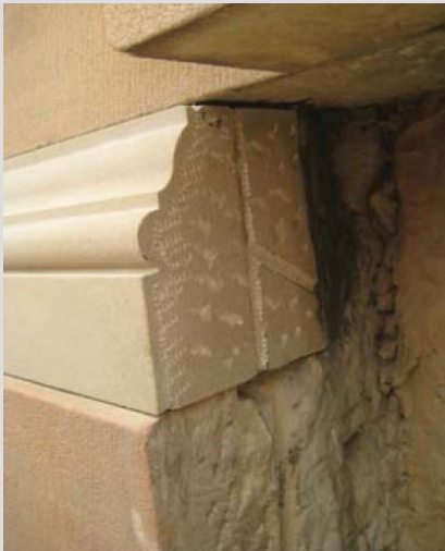
New indented stonework.
