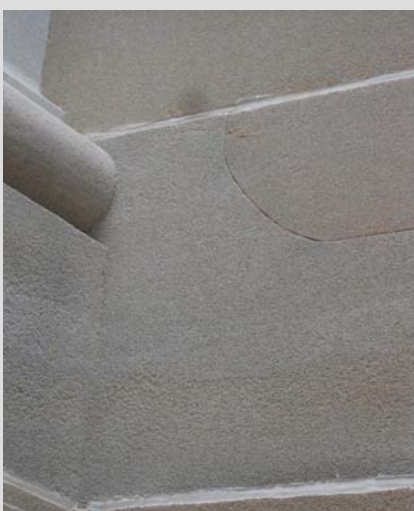
Hairline indent for small section of existing stone block.
