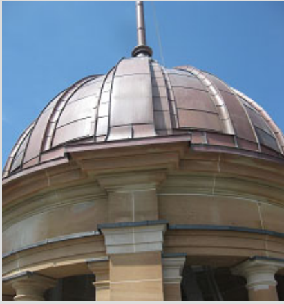
Introduced copper dome covering to protect original fragile stonework.
