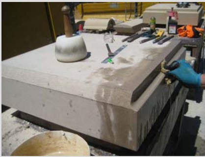
The replacement stone for the Clock Tower's Juliet 4 ton floor slab.
