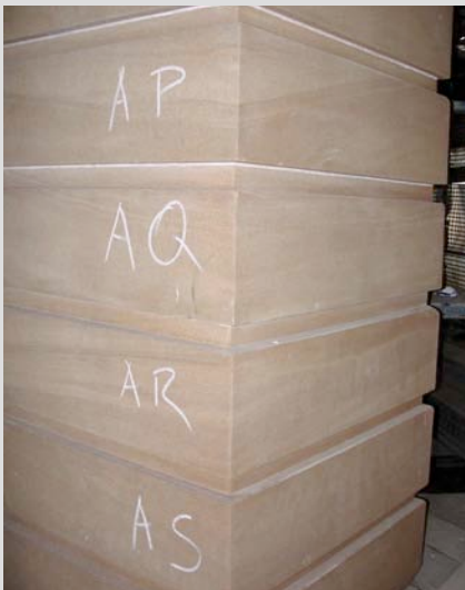
Every stone was individually numbered and entered onto a master drawing. Individual stones also had large-scale details drawn showing individual works.
