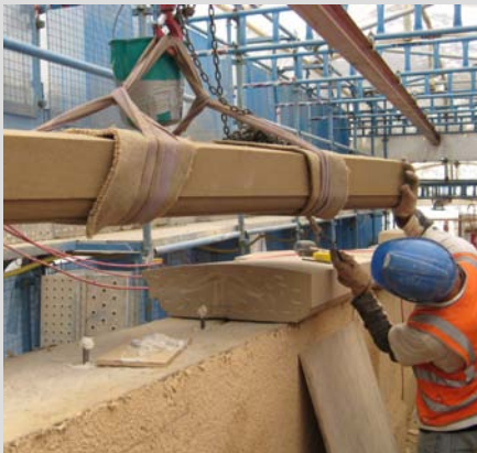
Stone block replacement for wall cappings.
