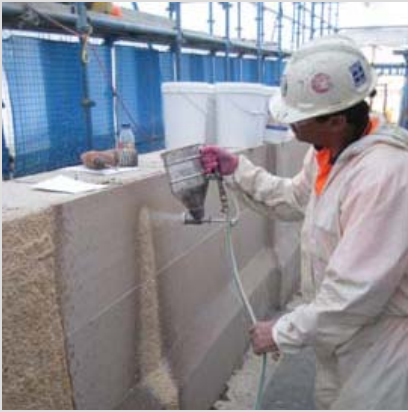
Paper-mache poultrice being applied to ramp up to Clock Tower.
