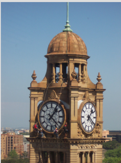
Consulting architects abseiling Central Station Clock Tower (2006).
