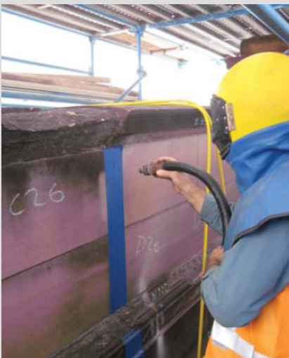
Cleaning of sandstone.
