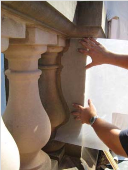
Masons ensuring accuracy by creating templates of existing stone profiles.
