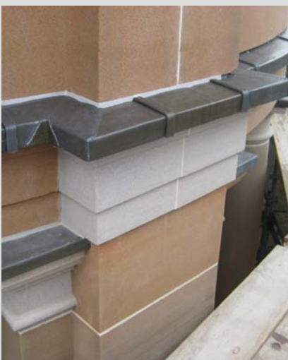
Protection of projecting stones through lead coverings.
