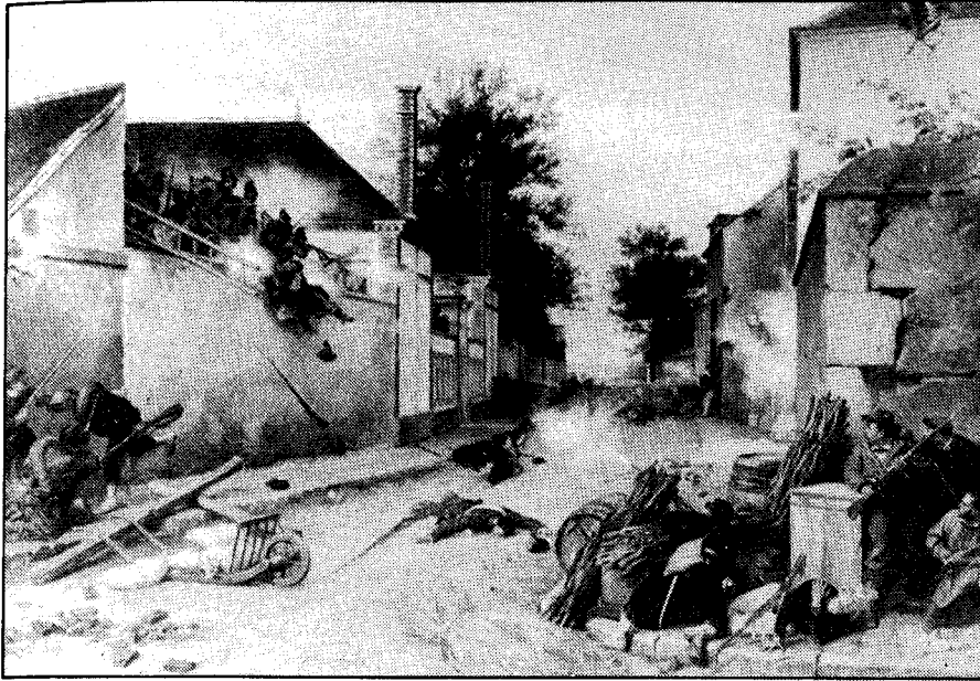
Barricade overturned at Châteaudun, 18 October, 1870.
