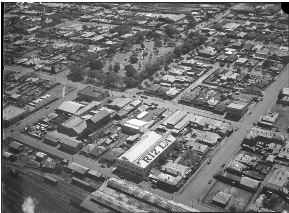
The factory stage 2 facing Roe St. and Perth Railway Station. This aerial photograph shows the bond store extending to James St. Evidently cigarette papers were being manufactured..
