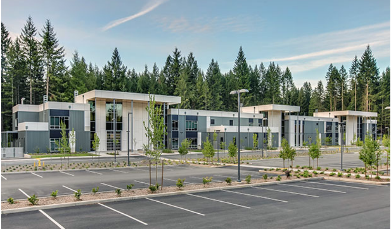
STEM High School in Lake Washington School District. Photo: Absher Construction Company. STEM is a sustainably designed 21-acre campus.
