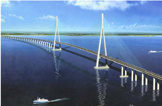
(c) Jiangsu Sutong Bridge
