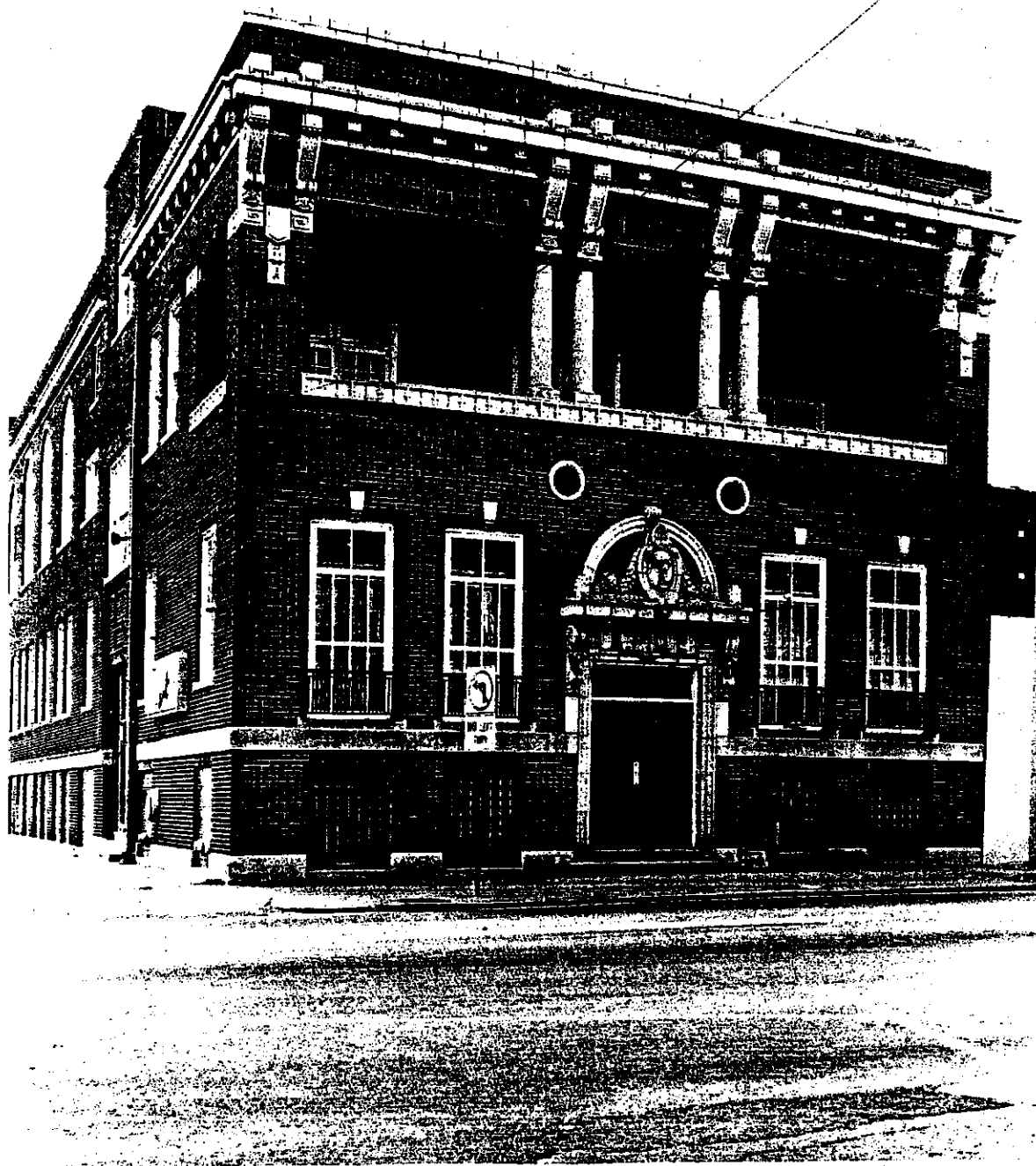
Figure 11. Ca. 1975, Murphysboro Elks Lodge. Note basement glass tile block windows and absence of original roof. Jackson County Historical Society, Photo Collection Album 30)
