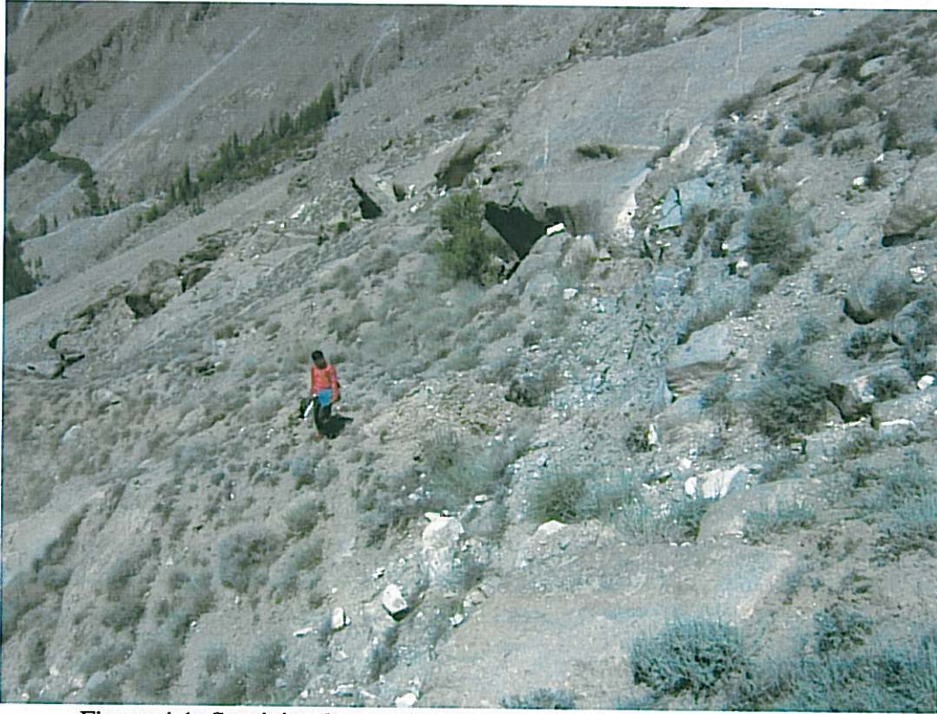
Figure 4.1: Semicircular crack with large displacements at backslope
