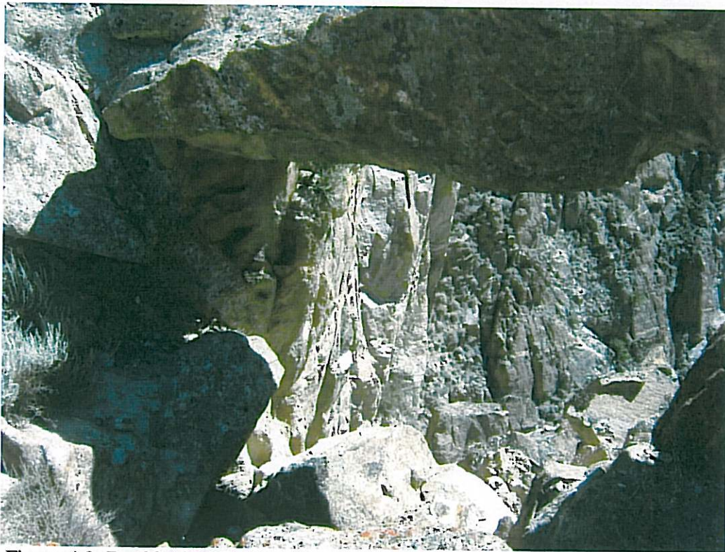
Figure 4.2: Boulder hanging dangerously on the widened crack at eastern margins
