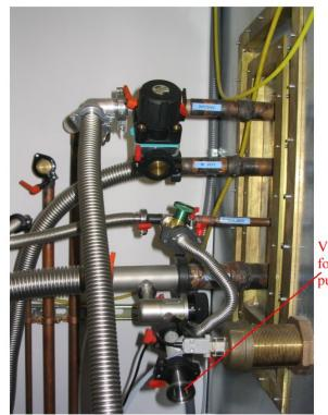
Vacuum connection for condenser & pumping lines
