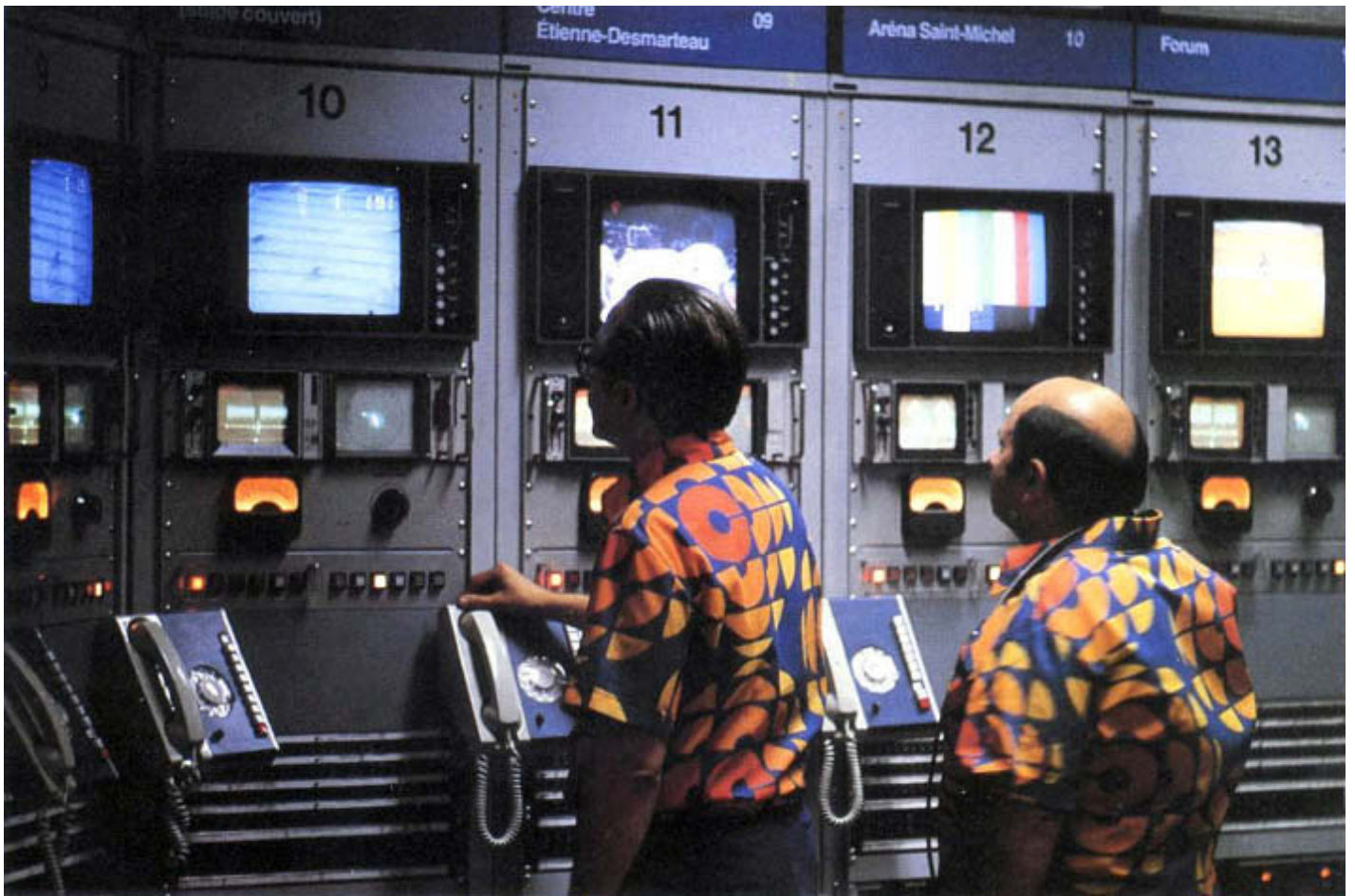
International pictures and sound were received at video and audio bays mounted on racks, from where they were ultimately broadcast.
