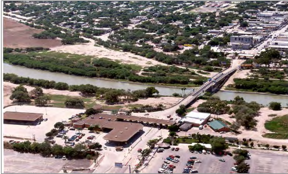
The United States is shown at the bottom of the photo. (Photo taken in 2000 before bridge replacement)
