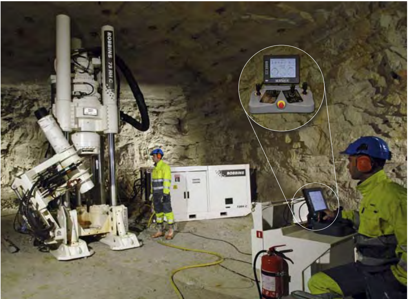
Figure 7: Robbins 73RH C with RCS control panel.
