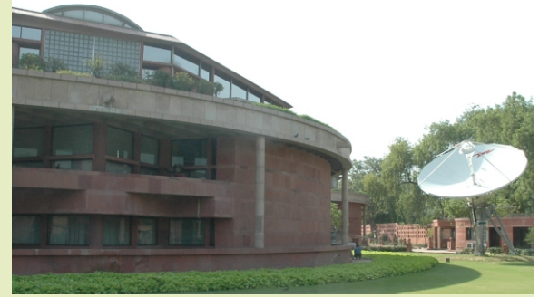
T.V. Antenna installed within Parliament Estate
