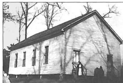
Old Goodsprings Cumberland Presbyterian Church building at Second Creek
