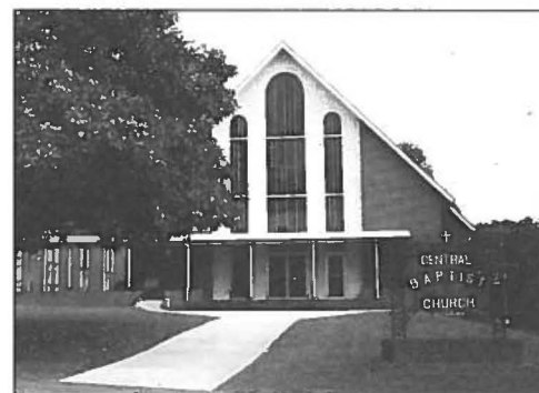
Central Baptist Church, Florence, Alabama
