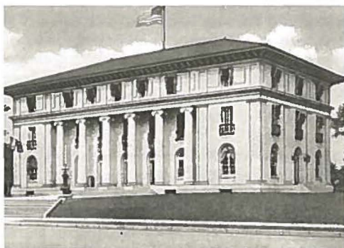
Florence Post Office and Federal Building
