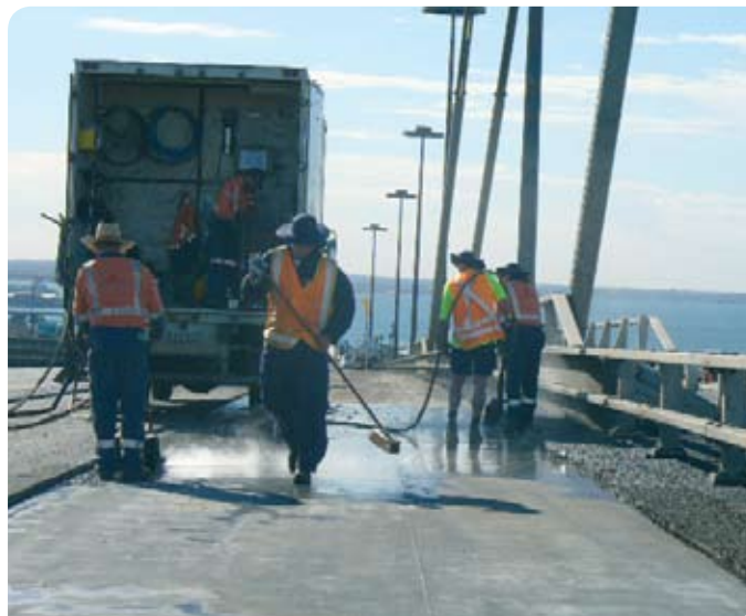
West Gate Bridge works
