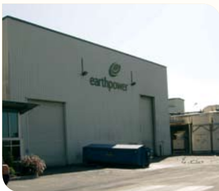
EarthPower; Food to Energy Facility
