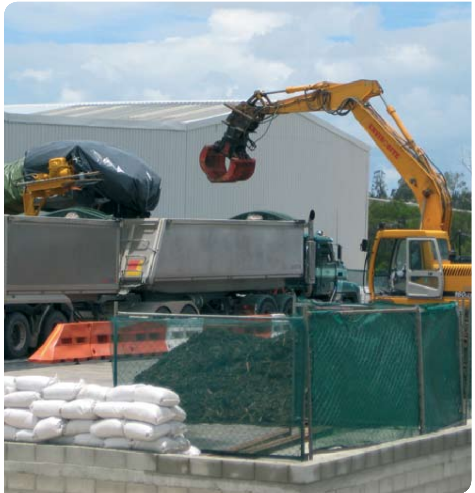
Loading solid waste using covered conveyor
