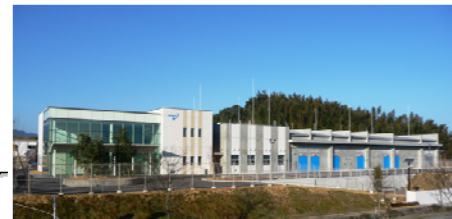
Hydrogen Energy Test and Research Center (HyTReC)
