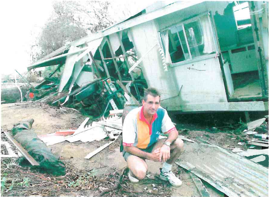
Severe flood damage at Black River, north of Townsville. (Photo courtesy of Queensland Newspapers)
