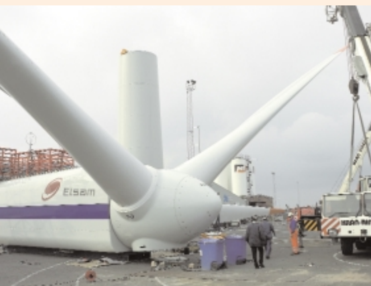
Construction of turbines for Horns Rev wind farm, Denmark
