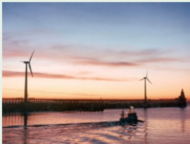
Blyth Harbour wind turbines, Northumberland coast.
