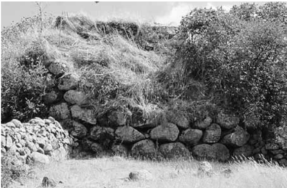
Fig. 73. Macomer, Nuraghe Porru: lato NO.
