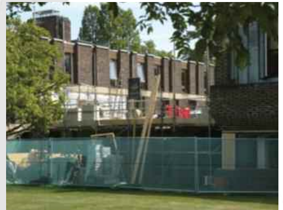
The new building nearing first floor level in August 2013.
