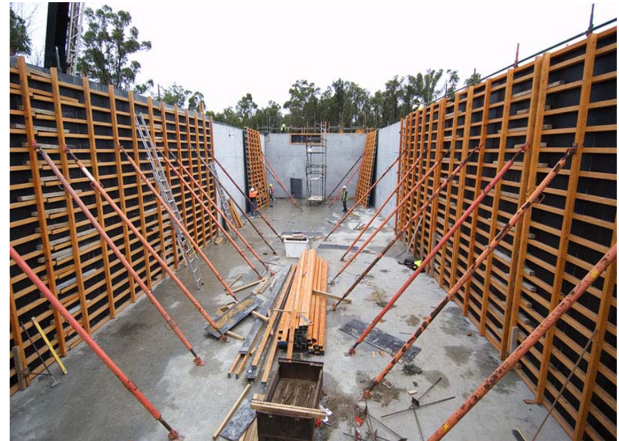
Construction of the new Sewage Treatment Plant, Wallacia
