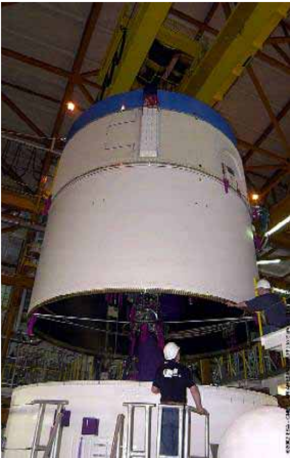
Kourou: erection of the Upper Composite in the Launcher Integration Building (BIL) © ESA/ARIANESPACE/Service optique CSG
