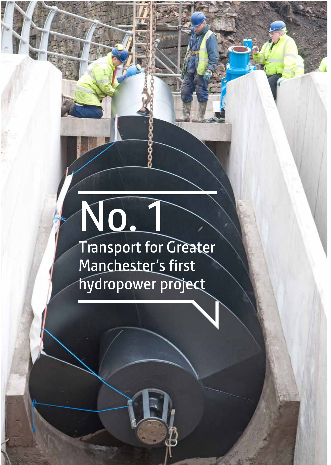
Installing the screw-turbine on the river Roch
