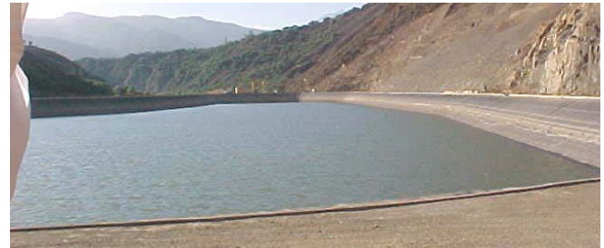
Reservorio San Diego
