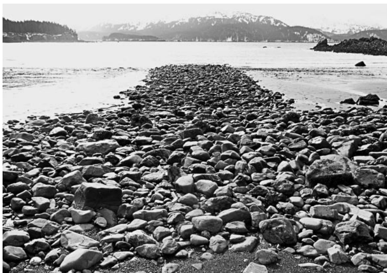
Fig. 1. The stone foundation of a Russian pier at the Coal Village Settlement (1855–1865), Kachemak Bay, Alaska
