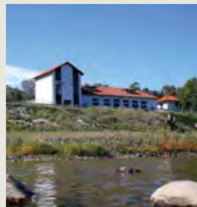
The Cotter Reservoir Pumping Station. MW
