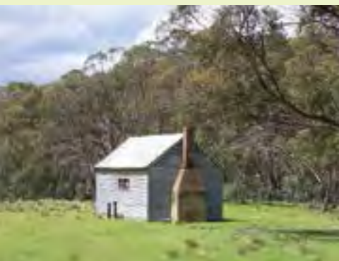
Horse Gully Hut on Mount Clear.
