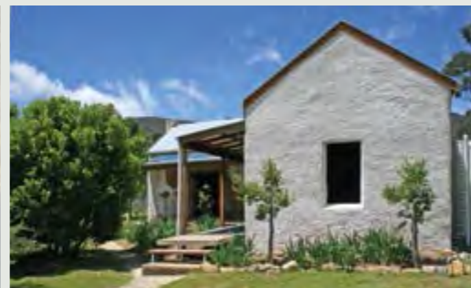
Rock Valley Homestead was fully restored after the 2003 bushfires.
