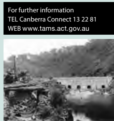
Cotter Dam construction. NLA
