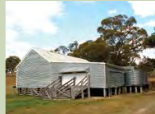
London Bridge Woolshed. MW
