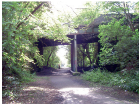
The steel road bridge
