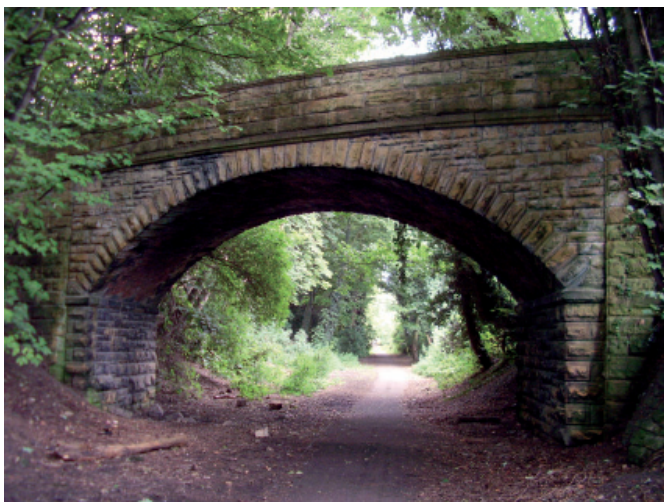
The stone railway bridge
