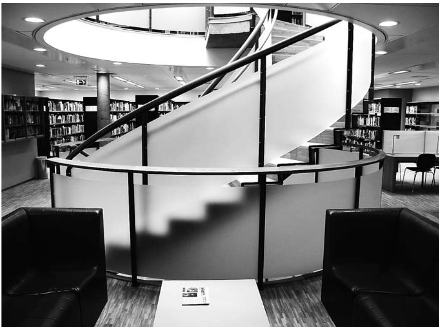
The spiral staircase is placed below the roof lantern.
