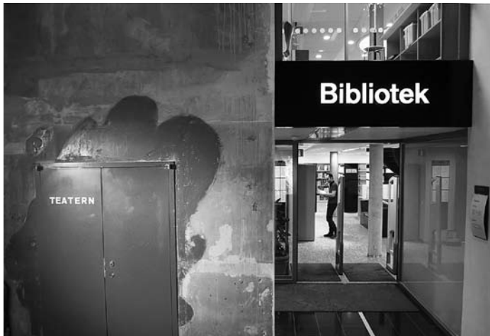
The new entrance to the library. Peter Celsing's original theatre entrance on the left.
