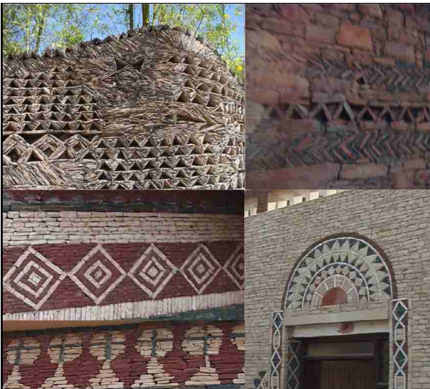
Figure 16 shows new and older (upper right) buildings of natural red, white and black "woven" stones and slate in Agadir. The two lower pictures show bricklaying patterns which can be ordered in Agadir's diy markets today. The patterns used are reminiscent of symbols of the Amazigh alphabet Tifinagh , which is at least 2,000 years old.
