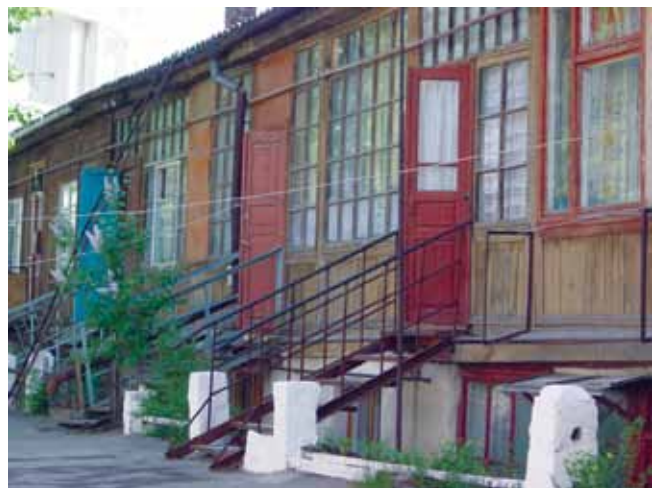
Backyard buildings of high preservation value
