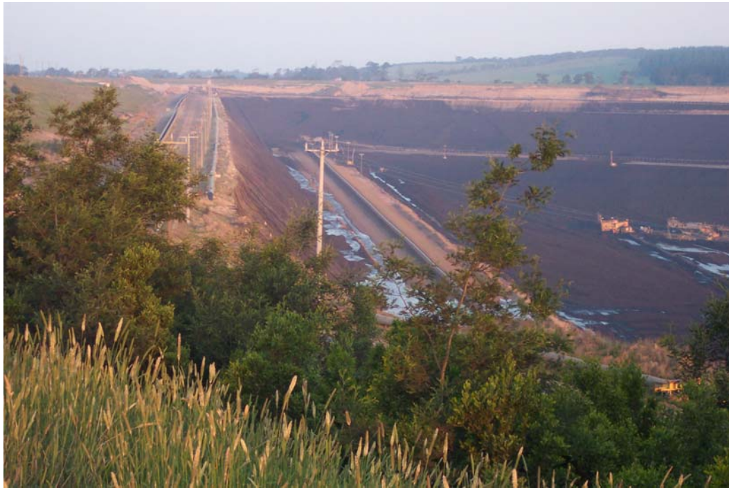
Figure 9: General view along, NE Batter, note the bends in the pipeline and the line of power poles
