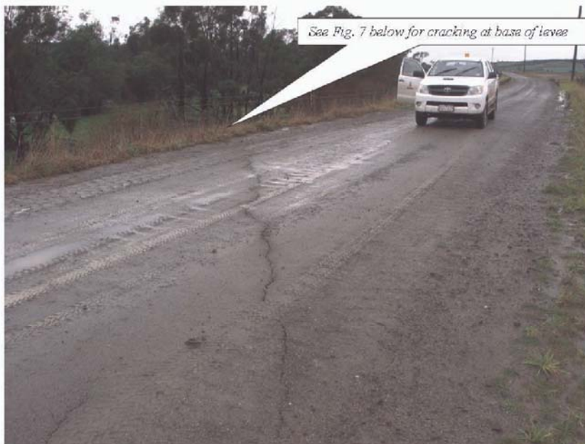
Figure 7 Cracking at base of levee Latrobe River Flood Plain
