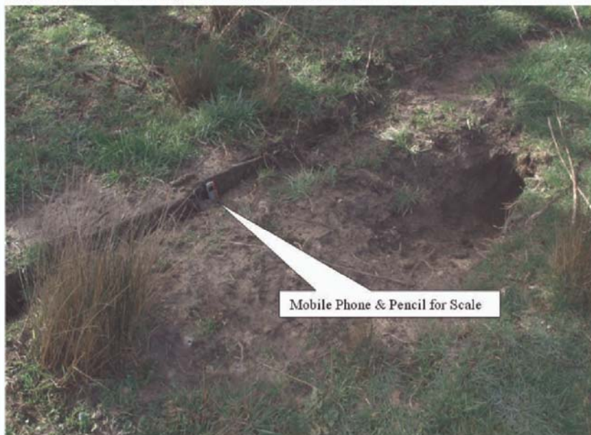
Figure 7 Cracking at base of levee Latrobe River Flood Plain
