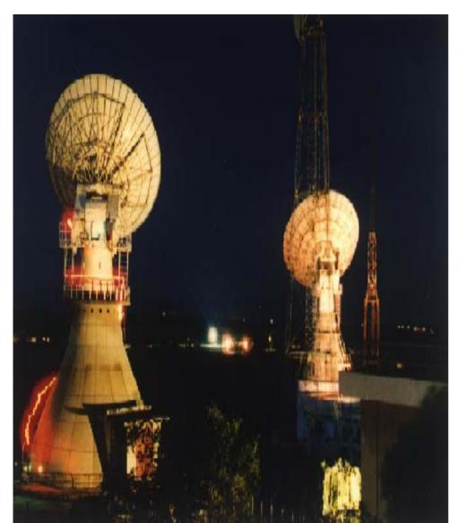
It includes Weinan Station, Xiamen Station and Instrumentation ships. It is equipped with C-band TT&C system, motion-limited station and telemetry reception station. It has ranging, angle measurement, telemetry and telecommand functions and is mainly used for GEO TT&C support.
