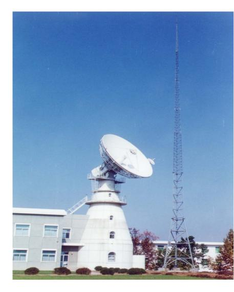
It includes Weinan Station, Xiamen Station. Qingdao Station, Nanning Station, Kashi Station, mobile stations and instrumentation ships. USB is the main equipment. It has ranging, velocity/angle measurement, telemetry, telecommand, voice communication and TV transmission functions, and is mainly used for low/medium orbit and manned spacecraft TT&G support.
