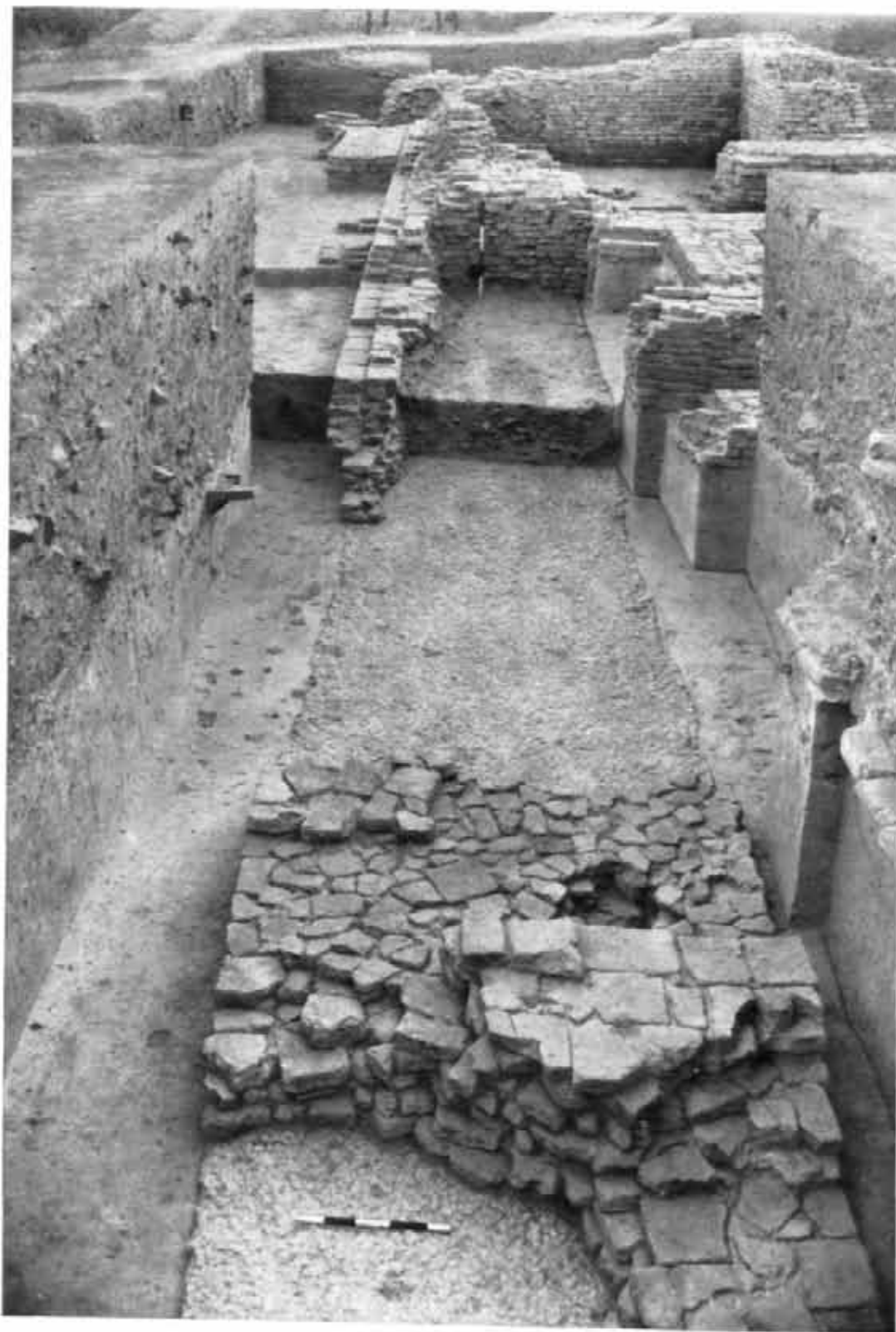
Bhitari : damaged eastern wall. See p. 47
