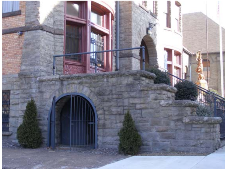
Detail, bathhouse entrance under 1889 section.
