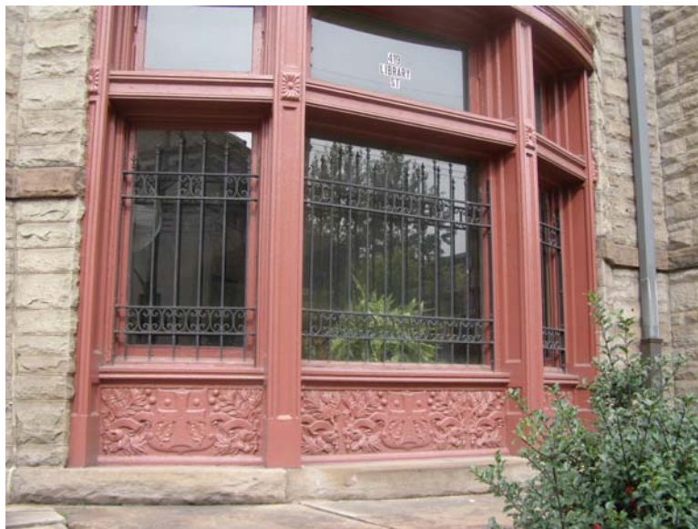
Detail, cast iron bay window, 1889 section.
