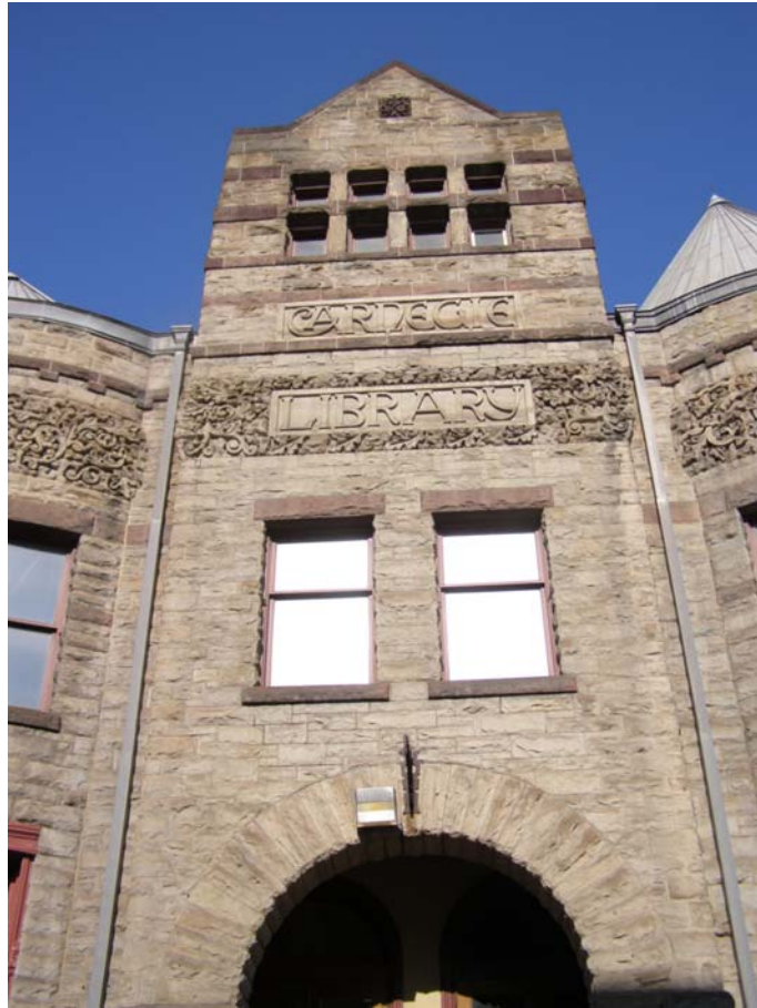
Detail, entrance tower to 1889 section.
