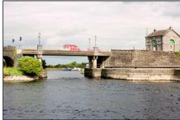
Navigation channel and lock house at Shannonbridge.
