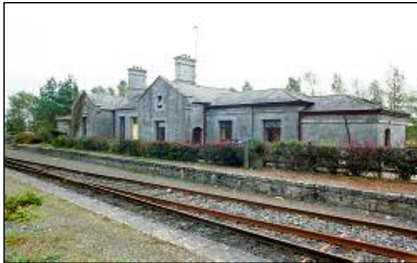
Knockcloghery Railway Station.
