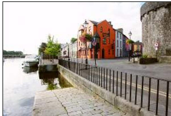
Athlone Quay and site of old town bridge.
