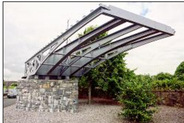
Section of former bridge over navigation channel.
