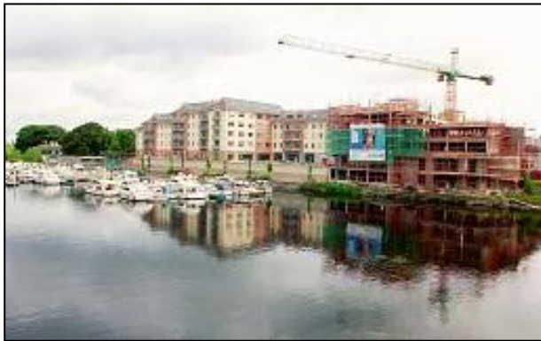
Top: Athlone Woollen Mills after fire in 1940 (O'Brien 2002). Bottom: apartments on the site of the mills, 2003.
