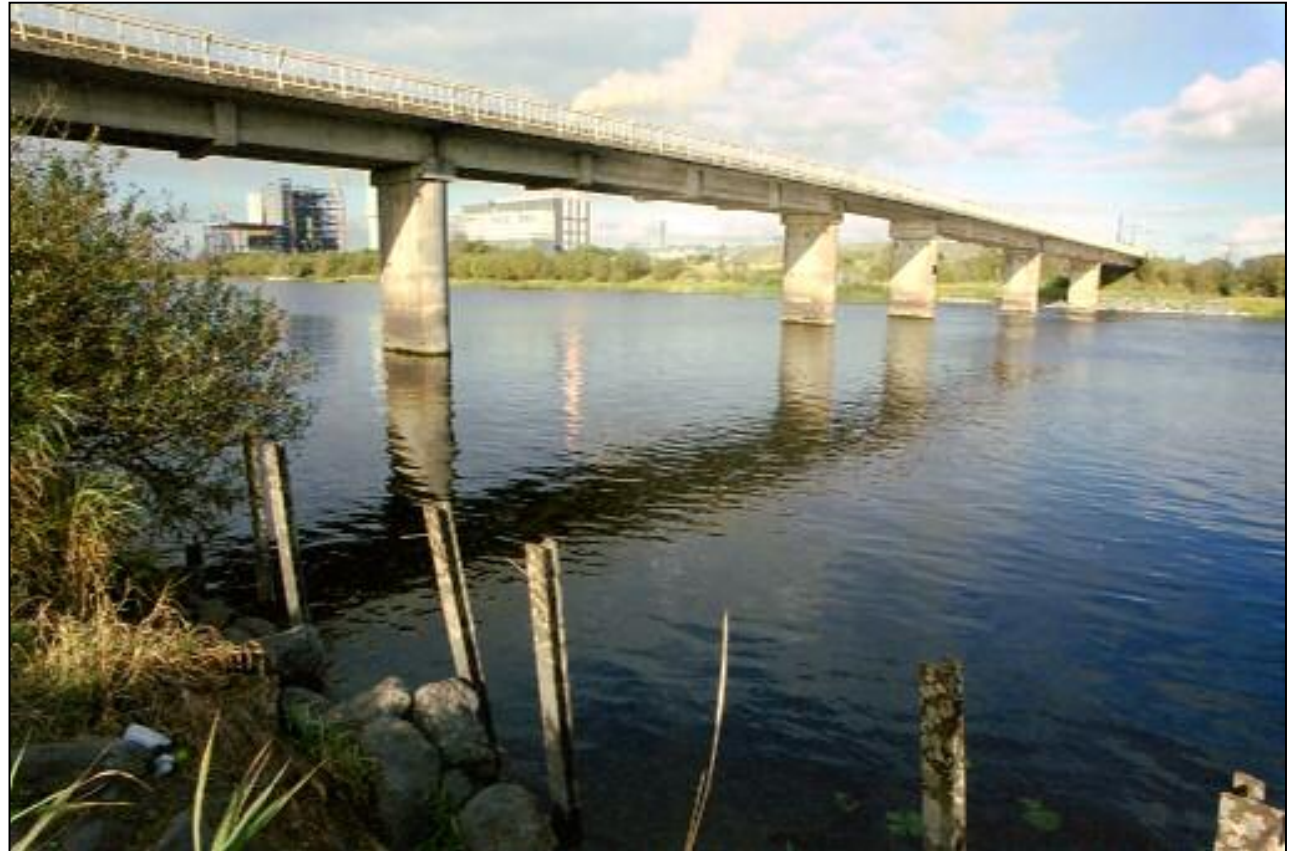
Peat railway bridge over Shannon, south of Shannonbridge power station.
