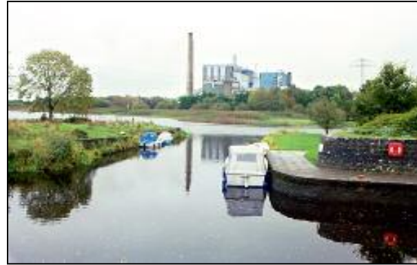
Lanesborough Power Station.
