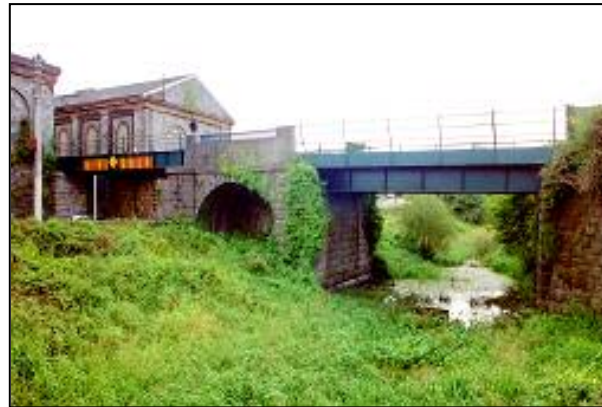
Railway bridge at north end of former Athlone canal.
