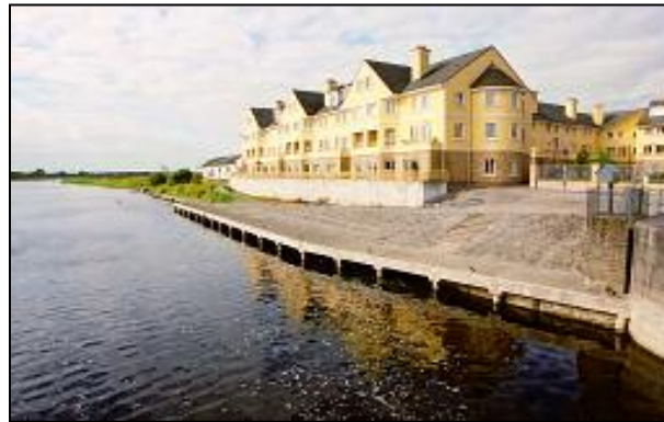
Top: Demolition of former distillery adjoining Athlone lock (O'Brien 2002). Bottom: the same scene today.
