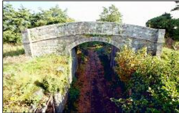
Kylemore Bridge, Ballinasloe Canal.
