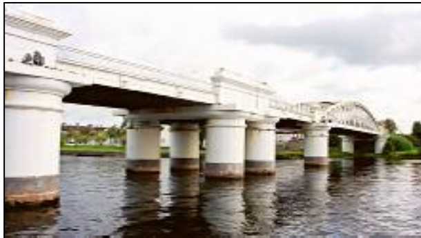
Shannon railway bridge, Athlone (1851).
