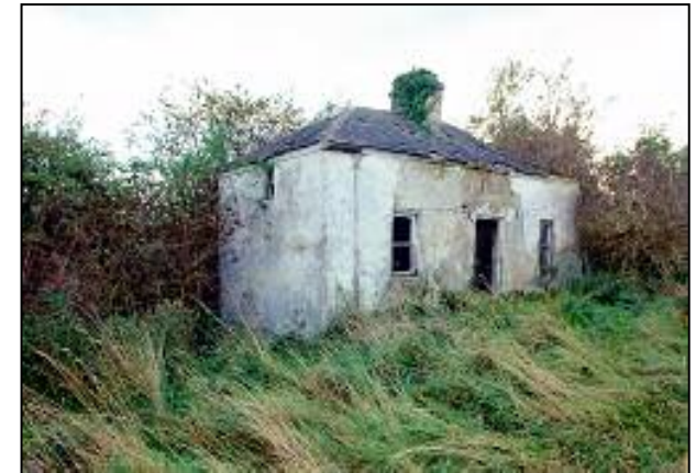
The derelict lock-keeper's house at Fanning's Lock.
