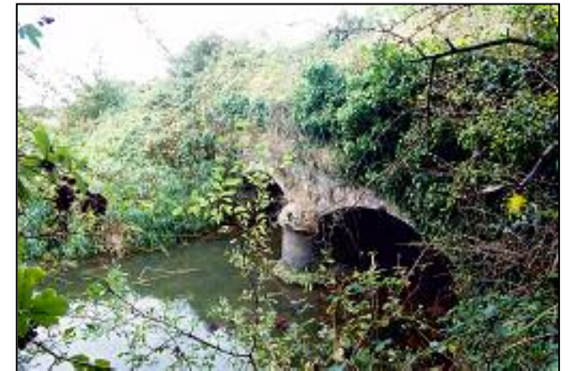
Canal aqueduct over Cloonascragh River.
